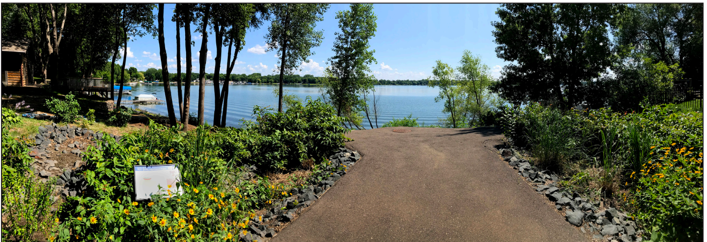
In Lindstrom, new or rebuilt city streets are made narrower when possible — a strategy that reduces stormwater runoff and cuts city maintenance costs. Linden Street was made narrower where it dead-ends at South Lindstrom Lake. It’s flanked by a stormwater treatment system that includes rain gardens.
